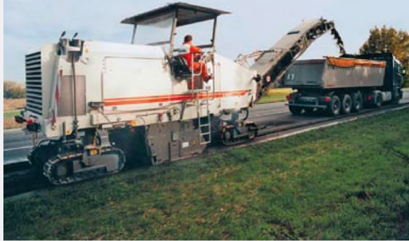
Large milling machine in operation
