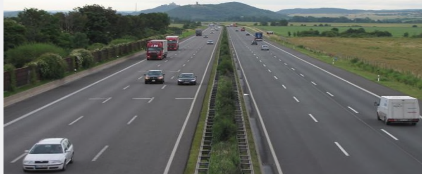
A4 State Highway in Germany (in use for over 18 years)
